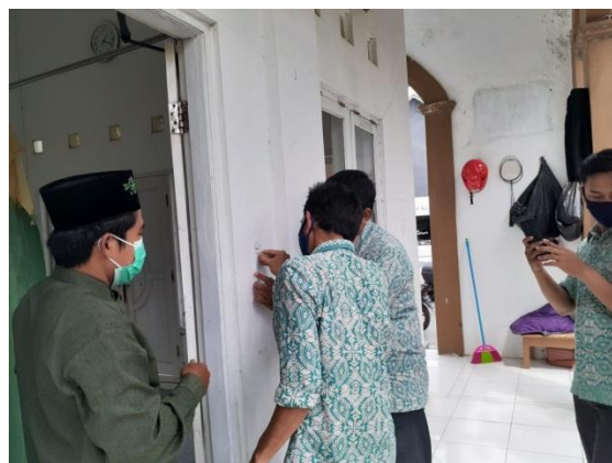
Gambar 6. Pemasangan Hand Sanitizer
